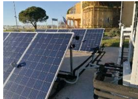
PV-T Panel Installation
