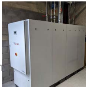
Cascade industrial sorption/propylene compression (30 kW cool)
