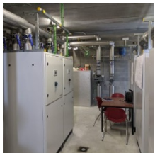
Facilities with hybrid chiller installed in solar driven plants
