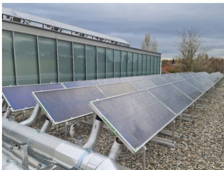
Solar cooling system installation in Spain
