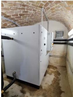
Geothermal gas-driven adsorption HP installation in a demo in Italy
