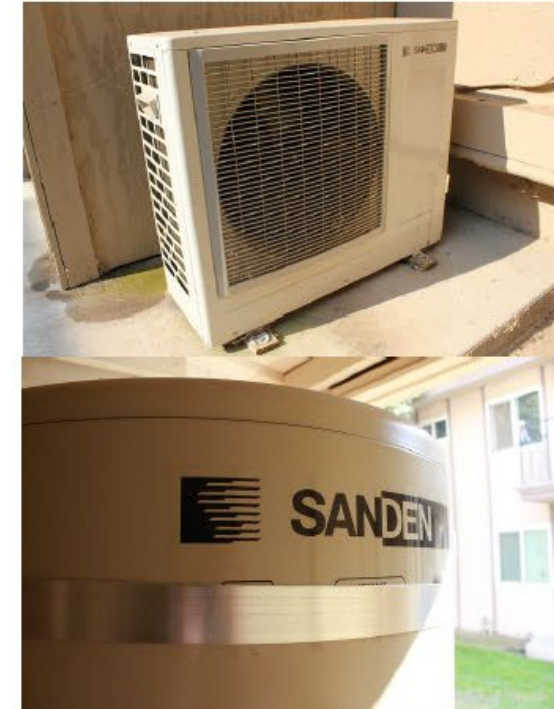
Low power HPWH (120V potential) with storage
