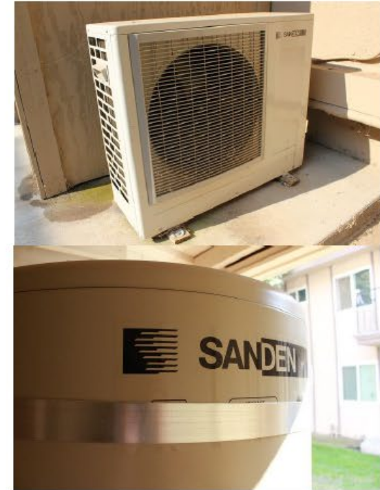
Low power HPWH (120V potential) with storage
