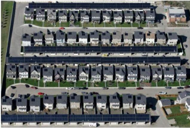
DRAKE LANDING SOLAR COMMUNITY Alberta, Canada
