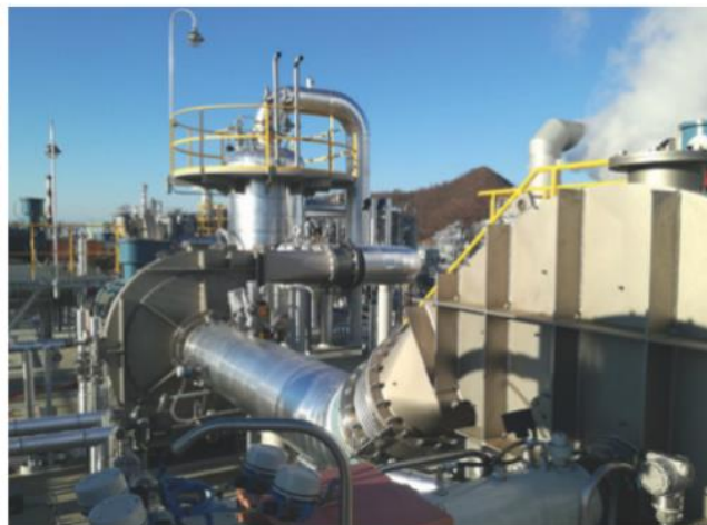
Figure 1: left: PILLER High Performance Blower, right: Multi-stage system in operation
