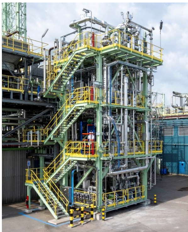
Figure 1: Heat transformer unit based on revolutionary Qpinch technology: commercial unit in Antwerp to demonstrate capabilities of technology as well as scale-up potential for wider Borealis operations and technologies
