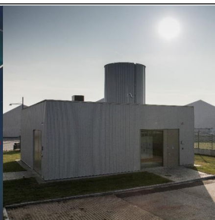
Figure 2 FlexHeat heat pump building and storage tank in front of cruise ship terminal building. Source: HOFOR
