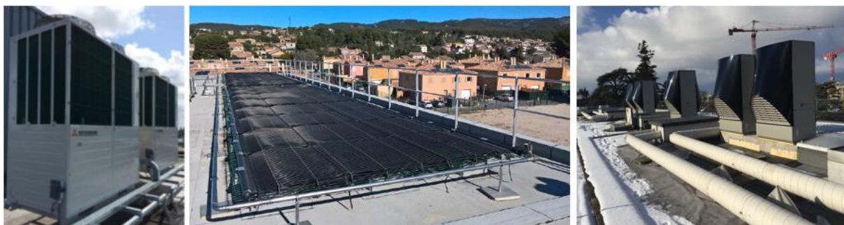
Figure 6: Examples of installed outdoor units or heat sources or HPs (source Suisse Energie and Giordano Industries)
