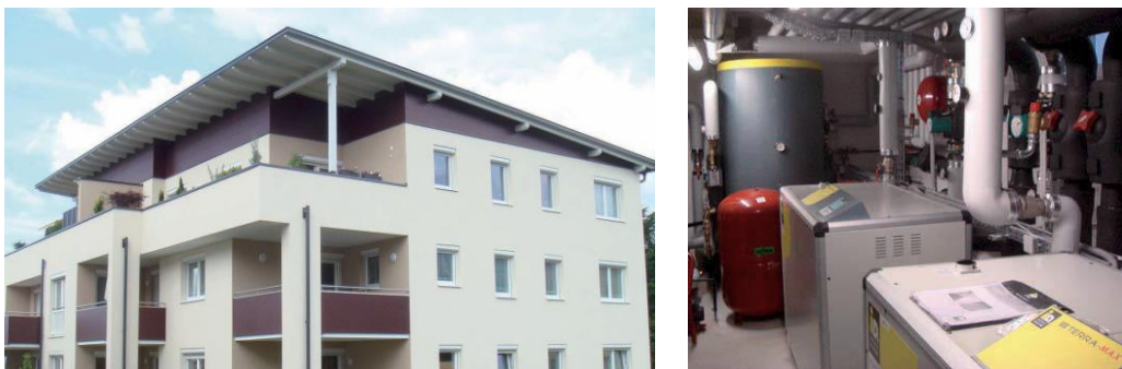
Figure 58: Pictures of the system in Villach (iDM Energiesysteme GmbH, 2017b)
