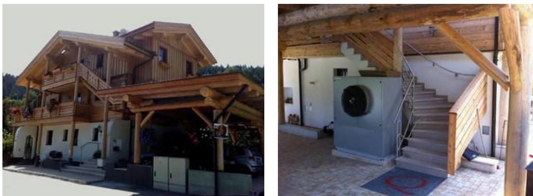
Figure 47: Pictures of the system in Bad Hofgastein (Glen Dimplex Deutschland GmbH, 2017)
