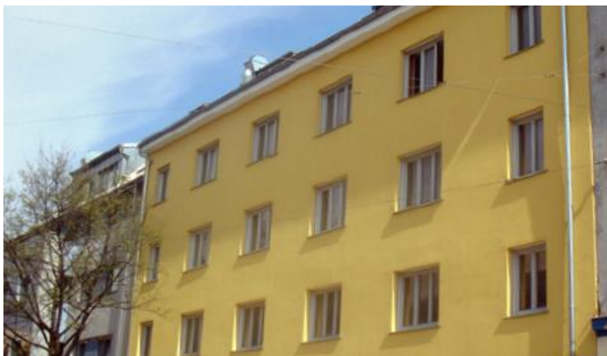
Figure 52: Picture of the building in Wien Simmering (Huber et al., 2014)
