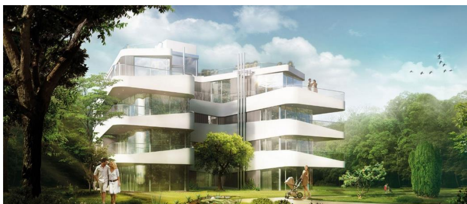
Figure 50: Pictures of the system in Vienna Residenzen Hohe Warte (Niederbrucker et al., 2016)
