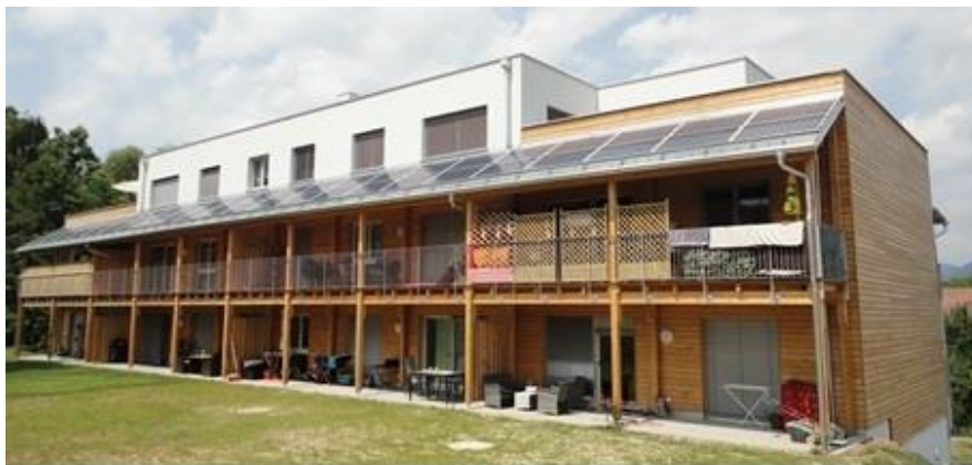
Figure 61: Building in Weiz (Hutter, 2016)
