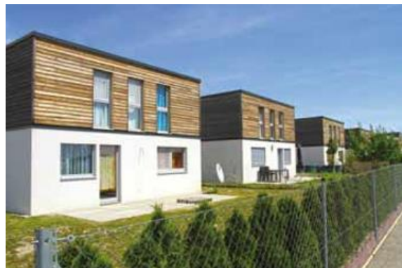
Figure 49: Pictures of the building in Vienna Podhagskygasse (Magistrat der Stadt Wien, 2012)
