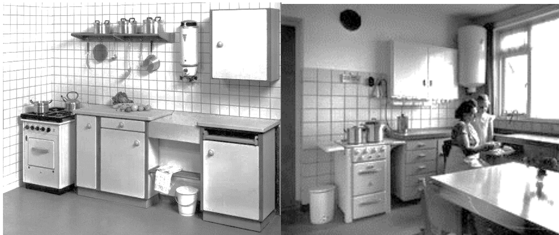
Fig: typically fifties and sixties, left: Kitchen with a geyser and right: Kitchen with electric storage water heater
