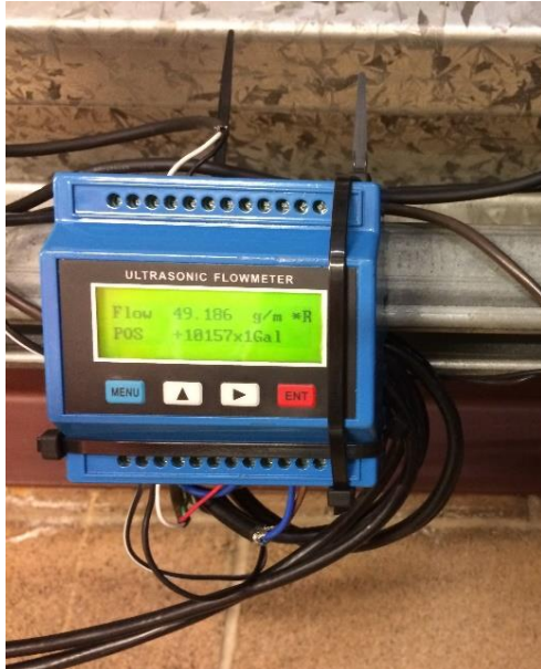
FIGURE 14 - GLYCOL LOOP TURBINE FLOW METER
