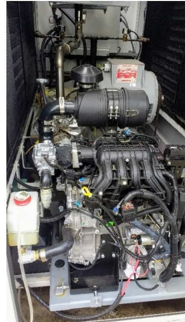
FIGURE 21 - ILIOS INTERNAL COMPONENTS
