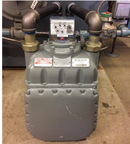
FIGURE 15 - ILIOS GAS FLOW METER
