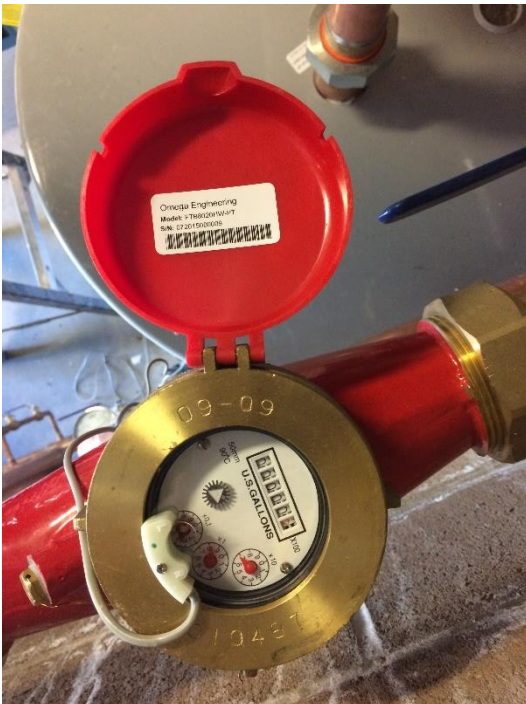
FIGURE 14 - GLYCOL LOOP TURBINE FLOW METER
