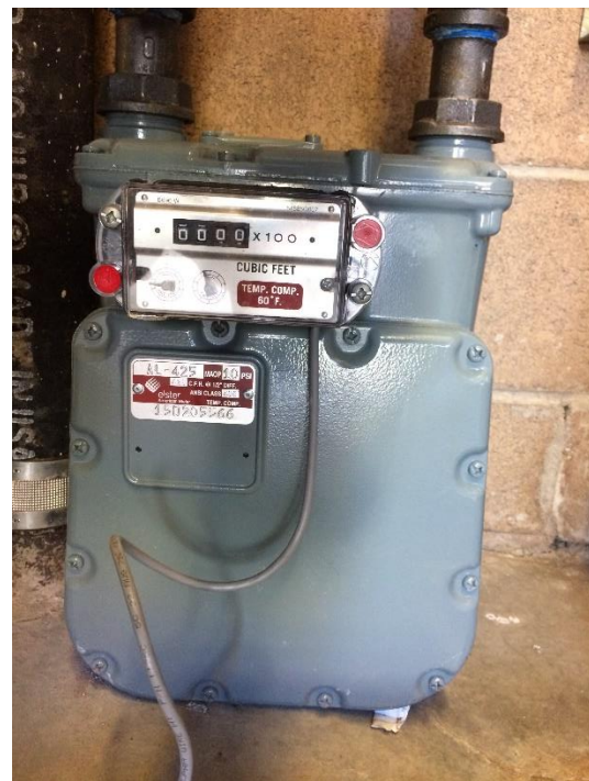
FIGURE 15 - ILIOS GAS FLOW METER
