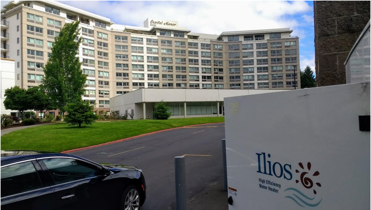
FIGURE 24 - CAPITAL MANOR TOWER POST-INSTALLATION
