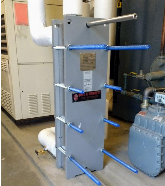
FIGURE 22 - DHW DOUBLE-WALL HEAT EXCHANGER
