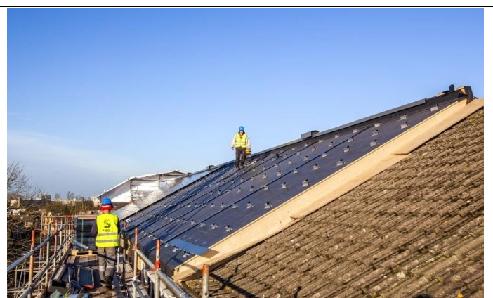
Installing PV panels –
