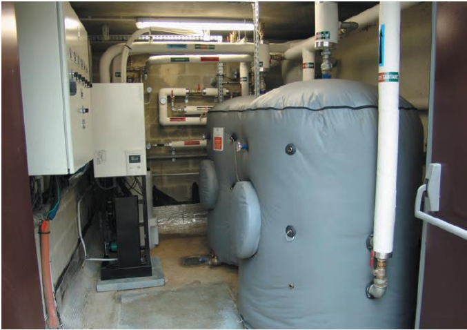
Substation with heat pump and two storage tanks 2 CORFLEX 1000L.
