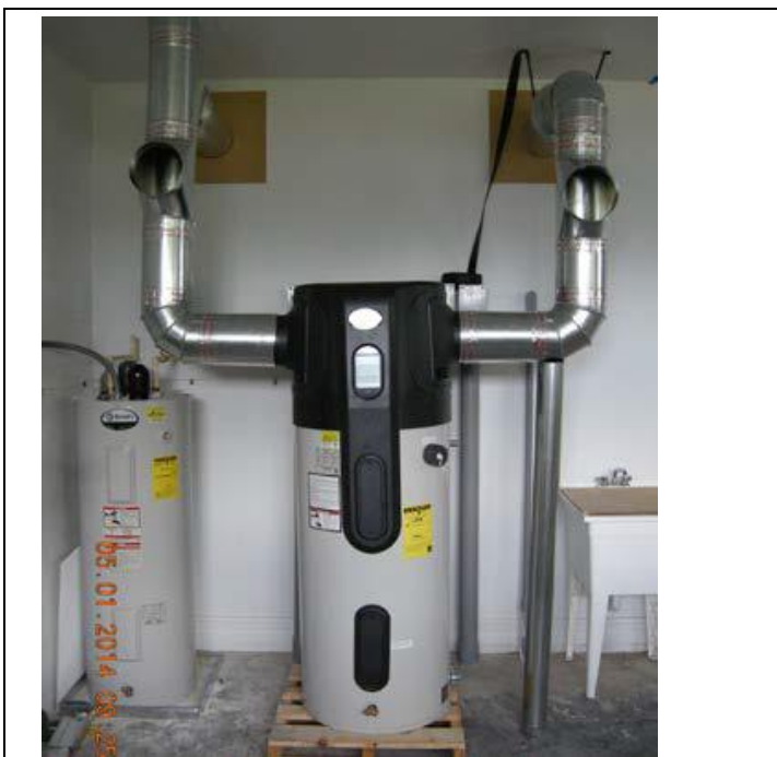
Heat pump water heaters were retrofitted with duct kits (shown without insulation) and manual directional dampers to study the impact of different airflow pathways.
