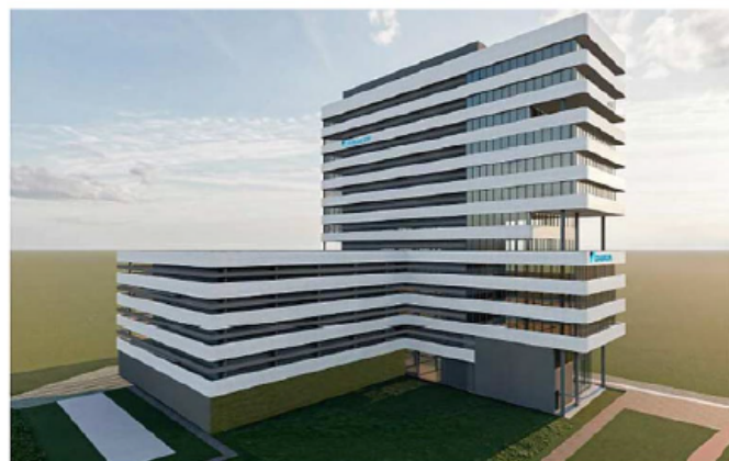
BELGIUM: Daikin Europe has begun construction of its new €140m EMEA Development Centre (EDC) in Ghent and announced further increases in heat pump production at Ostend.
