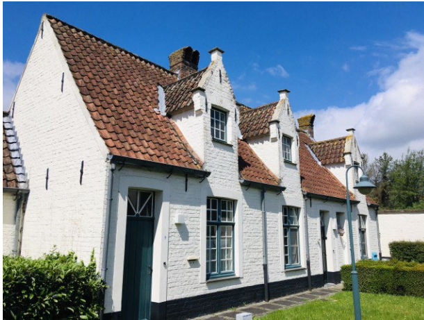
Figure 1: Building with 2 (out of 15) dwelling units
