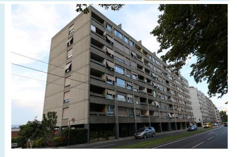
This existing MFH (multi-family building), built in 1972 in Geneva, contains 53 apartments over eight floors. It suffered no major envelope retrofit before this project and the total oil consumption amounted to 700 MWh/yr (for space heating and domestic hot water of its 4'049m<sup>2</sup> of heated area). (Photo credit SIG, CSD Ingénieurs SA)
