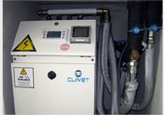
Complesso della Torre – Titanium steel ocean-thermal exchangers and a high efficiency water-to-water heat pump serving a flat
