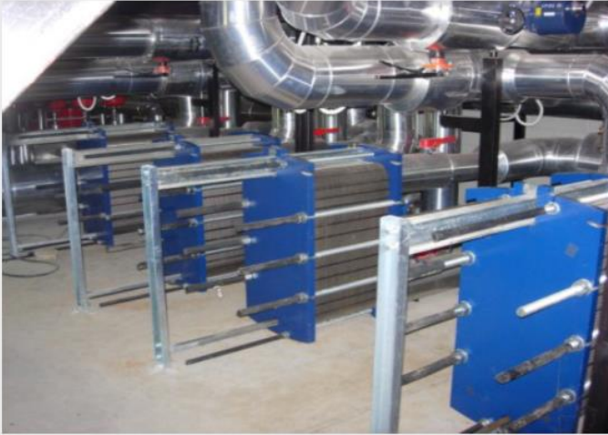
Complesso della Torre – Titanium steel ocean-thermal exchangers and a high efficiency water-to-water heat pump serving a flat
