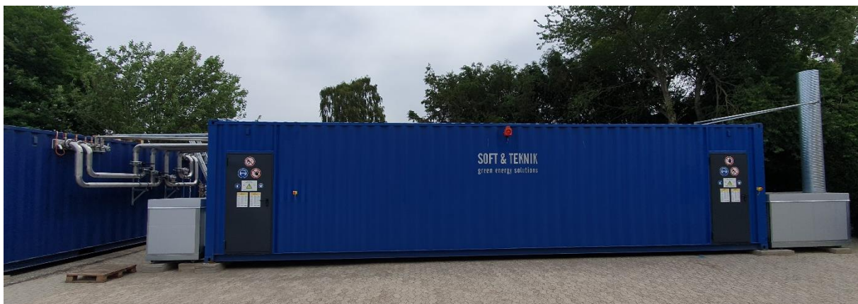
Figure 4-10: Pilot plant with 500 kW hydrocarbon heat pump from S&T installed at DTI (source: DTI).
