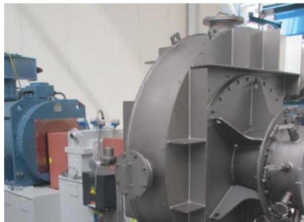
Figure 4-24 Piller high performance blower 10
