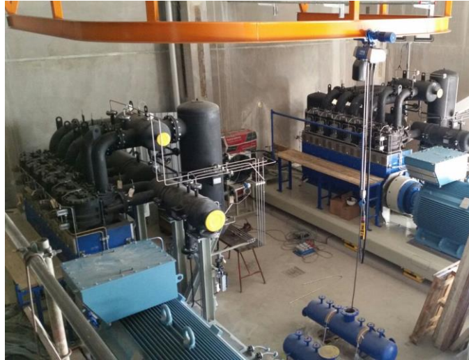
Figure 1: Steam compressors during installation at paper mill, Sweden.
