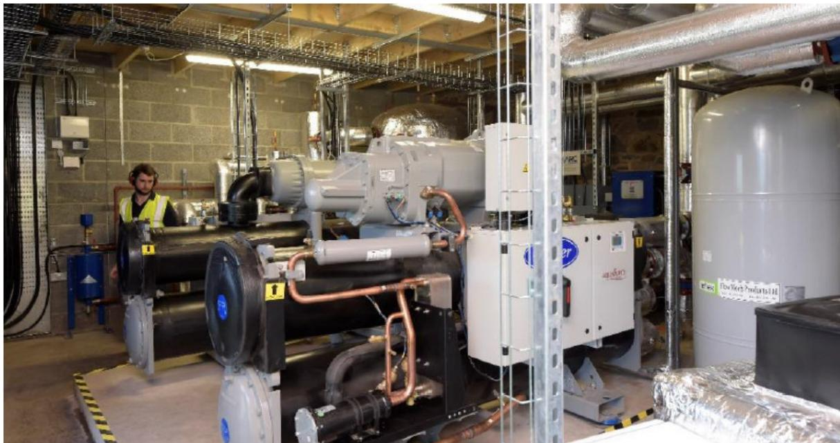
Figure 1: Sewage heat recovery system [3]
