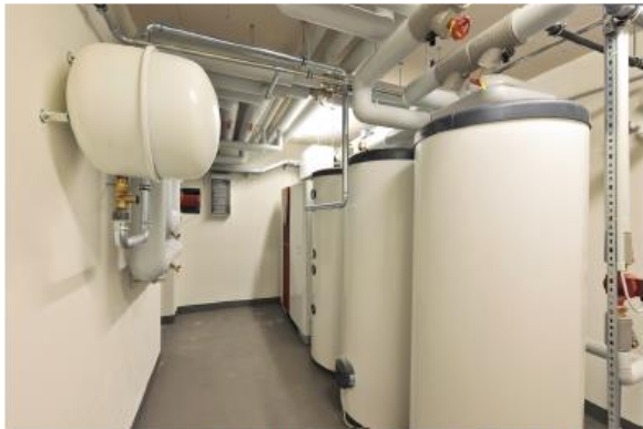
Technology room with 3 domestic hot water cylinders
