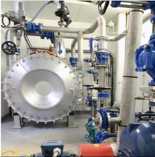
A process patented by Veolia, ENERGIDO recovers heat from wastewater. Wastewater, put in contact with a heat exchanger located outside the sewer system, conveys its energy to a fluid feeding the heat pump located within the facility. The latter returns the energy by producing water at the desired temperature (40° to 60°C) that feeds the heating network. Source [Veolia](#)
