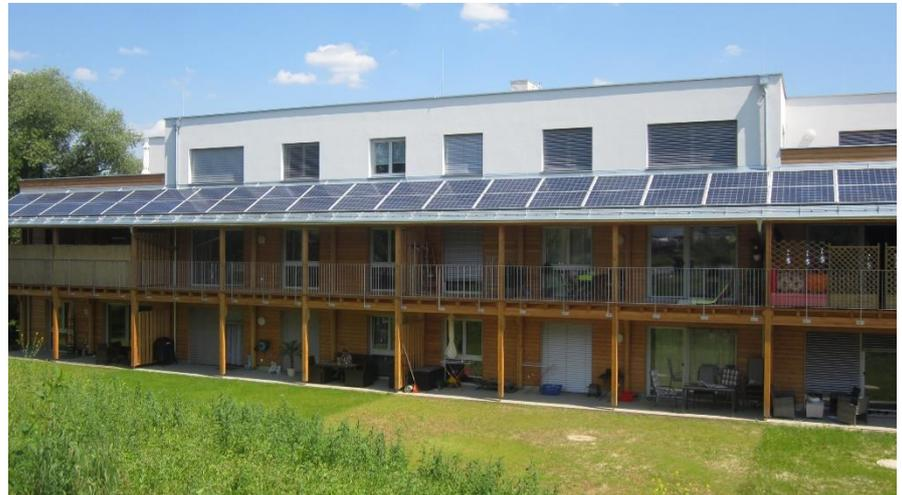
The construction of the MFH (multi-family building) which is located at Bärenthalweg 6 in A-8160 Weiz was finished in April 2015. The building is a wood frame construction which accommodates ten different apartments on three floors. The total area adds up to 1477 m<sup>2</sup>, whereof an area of 957m<sup>2</sup> is heated.
